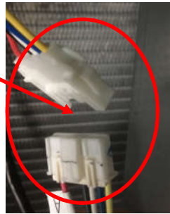
Disconnect fan motor harness
