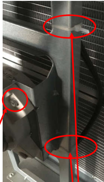
Unscrew the 4 bolts of the fan motor
